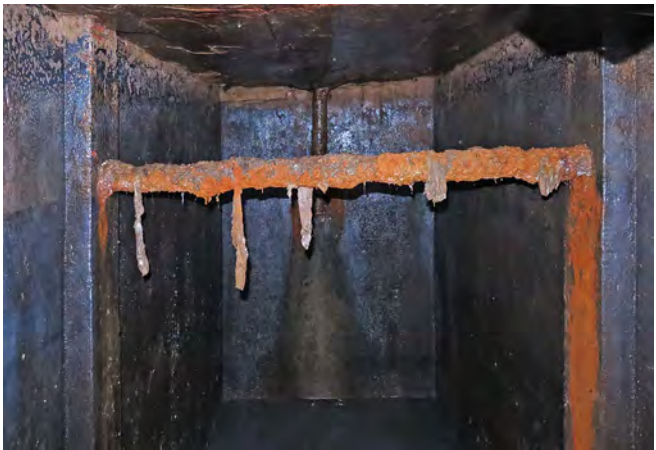
Inside the septic tank which appears somewhat narrower than an ROC post. Photo Clive Penfold
